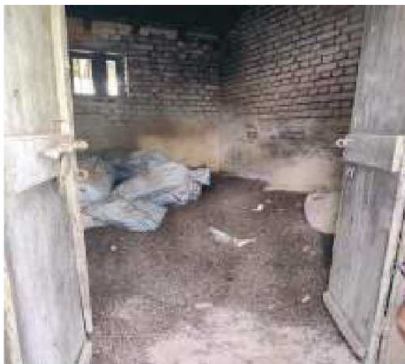
Photograph 3.3: Drugs kept in Muddamaal Room due to absence of dedicated storage facility
