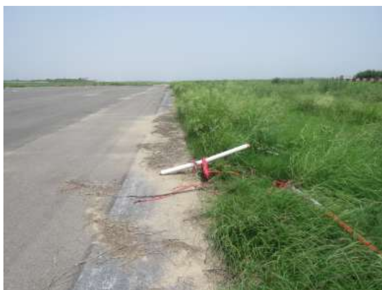
FIG 9: Location of Far Field Monitoring Antenna after the incident
