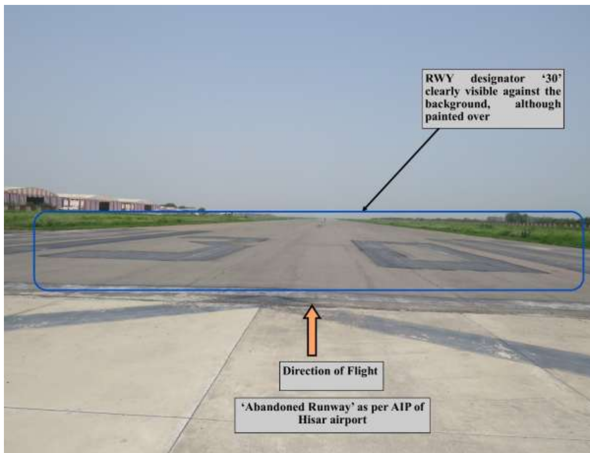
FIG 8: 'Abandoned Runway' portion ahead of RWY30
