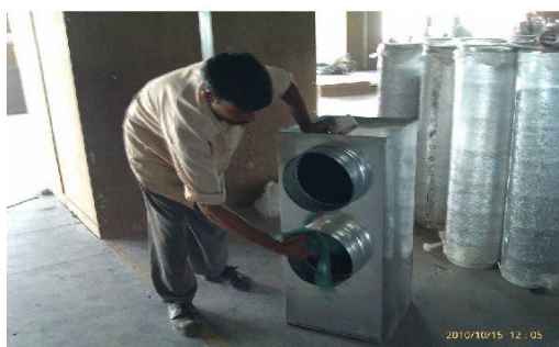
Ducts Wrapped with Plastic To Avoid Dust Plastic
