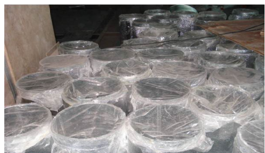
Ducts Stored with Properly Wrapped with
