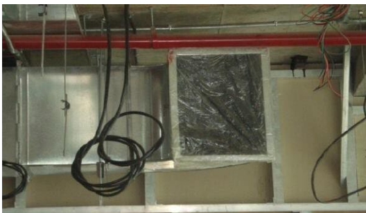
Ducts Wrapped With Plastic To Avoid Dust Wrapped with Plastic
