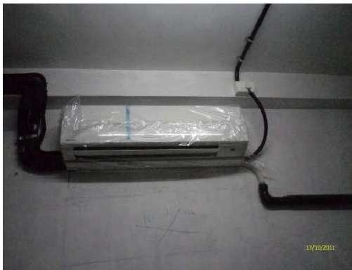
Equipment covered during Construction Phase
