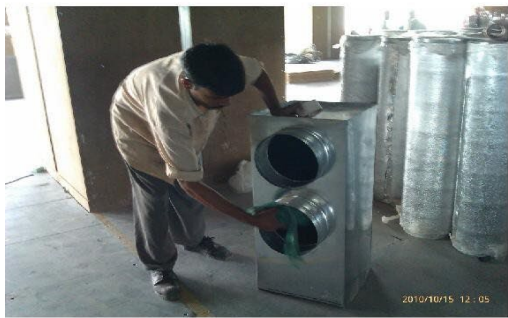
Cleaning Prior To Installation
