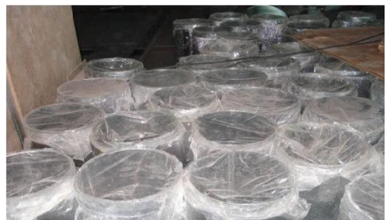
Ducts Stored with Properly
