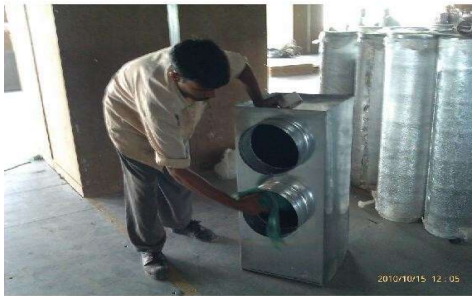
Cleaning Prior To Installation
