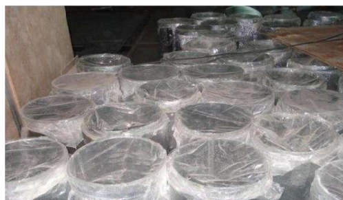
Ducts Stored with Properly Wrapped with
