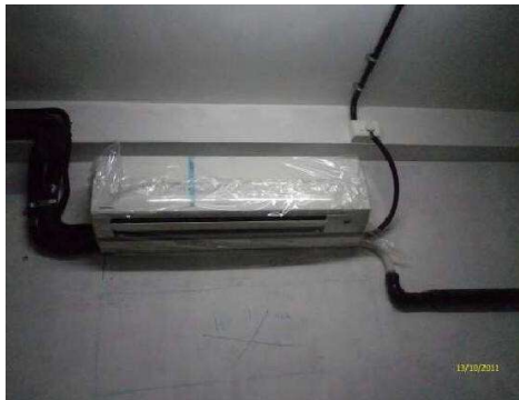
Equipment covered during Construction Phase
