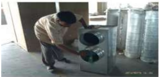
Cleaning Prior To Installation
