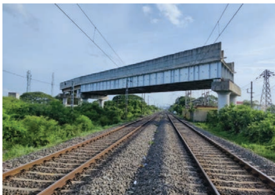
Incomplete Bridge Proper across the track at Acharapakkam Yard
