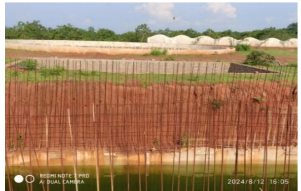
Picture 3.1.2: Construction going on for a Water park instead of plantation under 'Mahatma Gandhi Ausodhiya Aranya' Project (Date: 12.08.2024)
