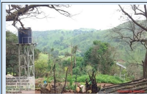
Photo 1: Solar energy-based water supply system at Suripada village of the Korukonda Block (24 HHs) (26 September 2024)
