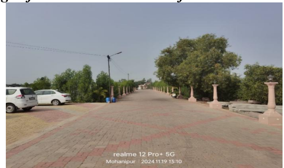
Picture 3.1.5: Construction underway for Swami Narayan Mandir Trust (Date: 19 November 2024)
