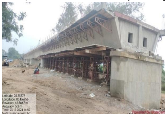
Picture 3.2.2: Bridge over River Kuanria without approach road (Date: 23 December 2024)
