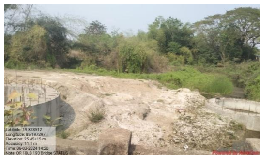
Picture 3.2.2: HL Bridge over Hatinallah
