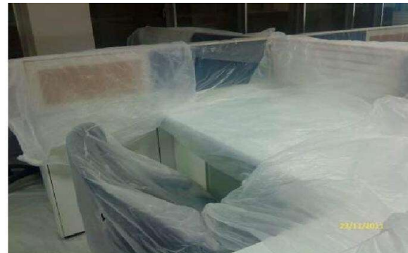
Equipment covered during Construction
