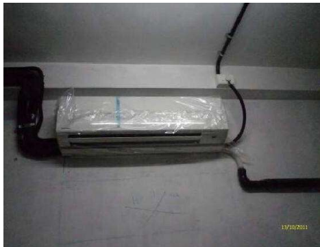
Equipment covered during Construction Phase
