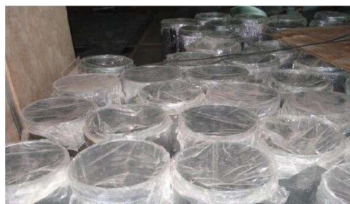
Ducts Stored with Properly Wrapped with
