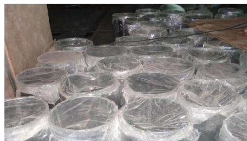
Ducts Stored with Properly Wrapped with
