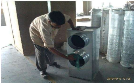
Cleaning Prior To Installation
