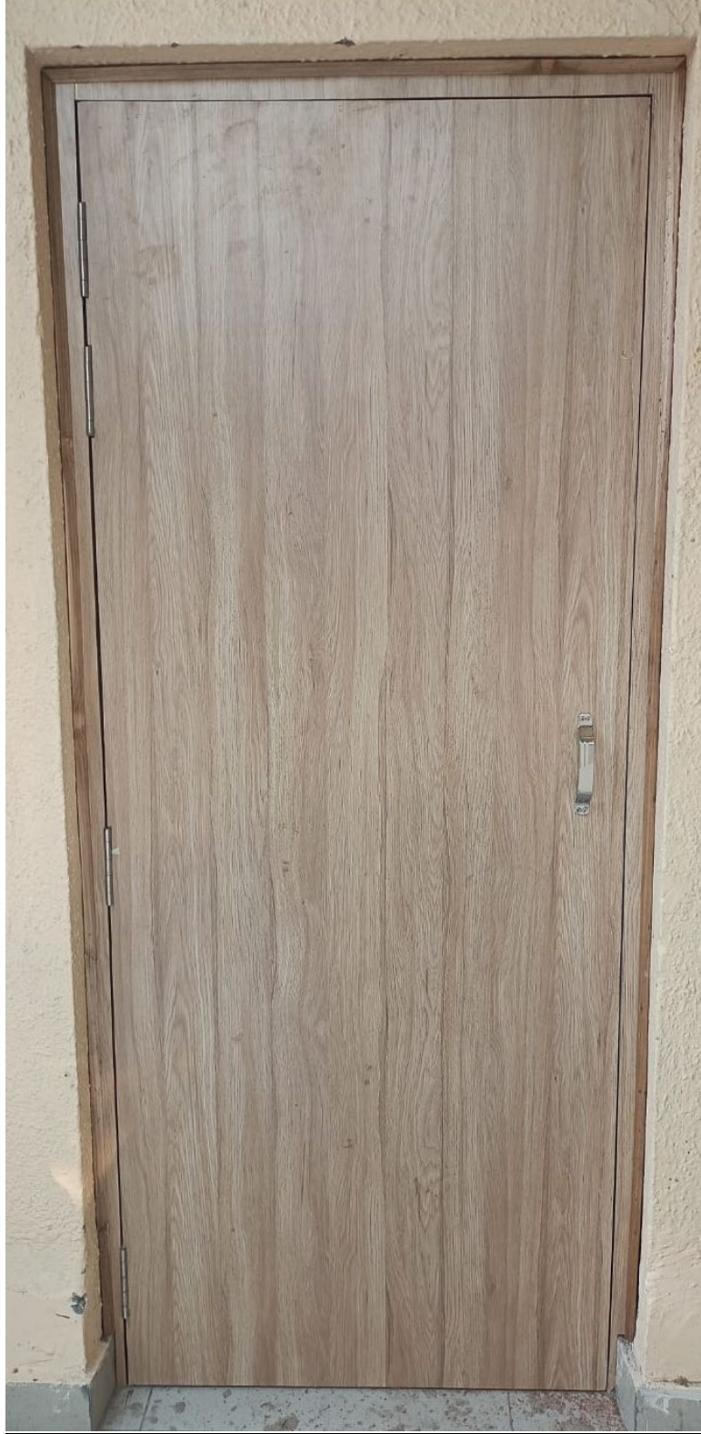
Outer side of Balcony gate
