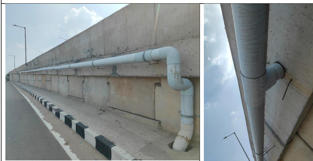
Alternatively: Long pipe slopped along ramp with connection with drainage spout & vertical take down pipe and connected to main drain
