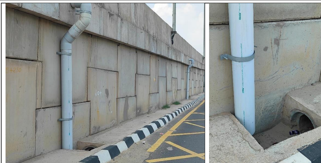
Takedown pipe at interval with 300mm Dia. HP in separator and cross connection to side drains.
