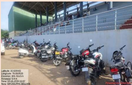
Lack of parking facility
